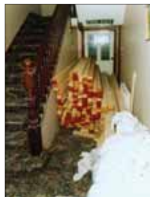
Figure 9: A blocked corridor with incorrect signage
