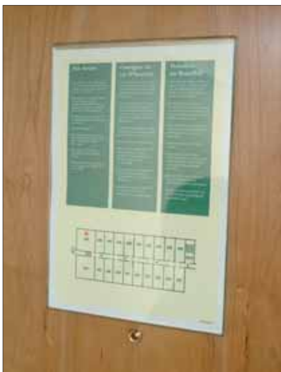
Figure 61: A typical bedroom fire action notice
